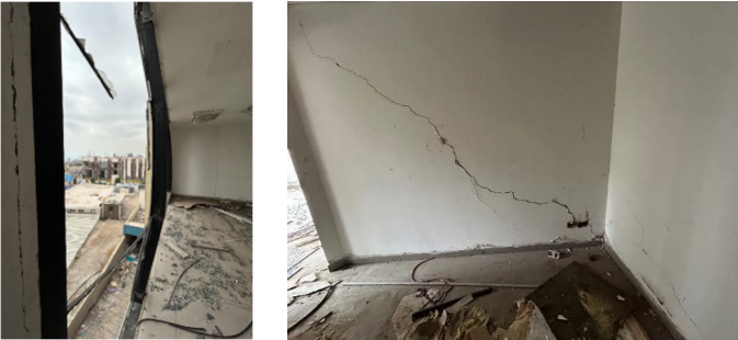
Figure 6. Post-2010 Reinforced Concrete Building Non-Structural Damage
