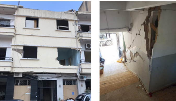
Figure 5. 1950's Reinforced Concrete Building Non-Structural Damage
