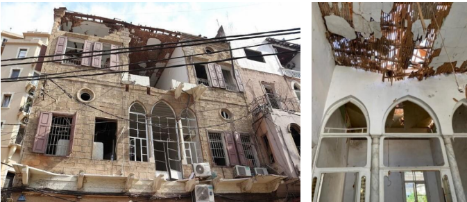
Figure 4. Natural Stone Masonry Historical Building with Partial Collapse
